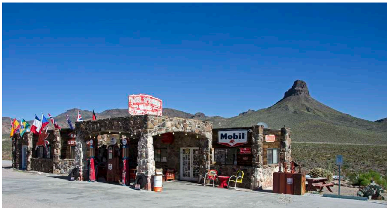
Title: Cool Springs in 2008 after restoration.
