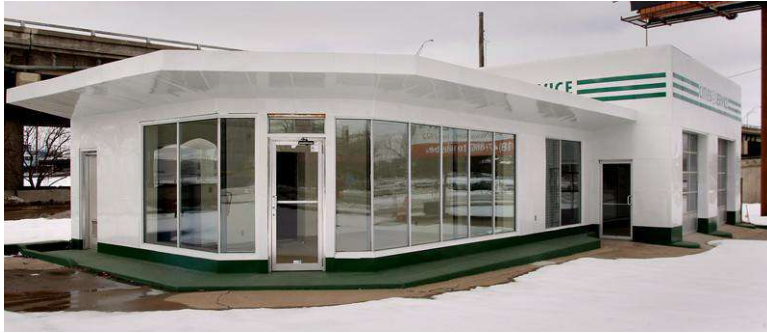
Title: The Cities Service Station #8, at 1648 SW Boulevard in Tulsa, Oklahoma, was built in 1940 and was listed on the National Register of Historic Places in 2011.
