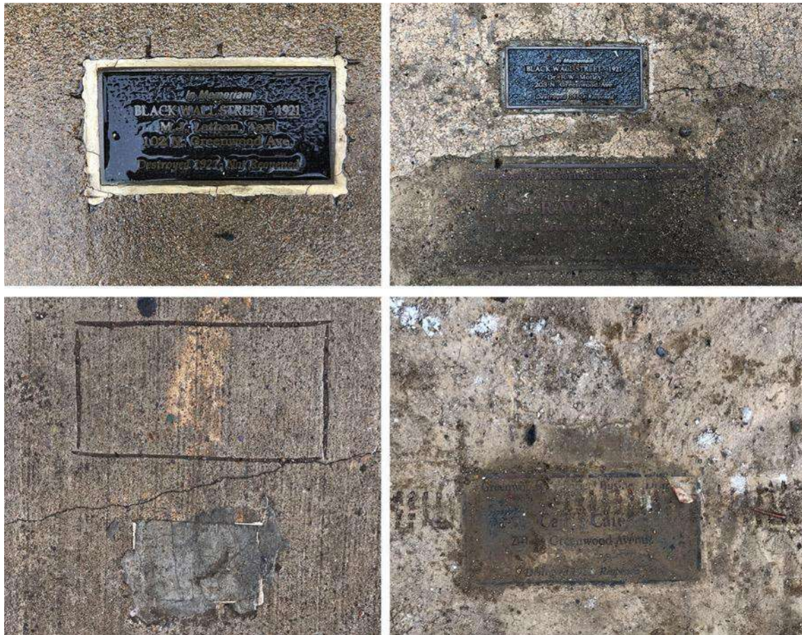
Image C-25: Commemorative Plaques in the Greenwood District, missing or damaged.
