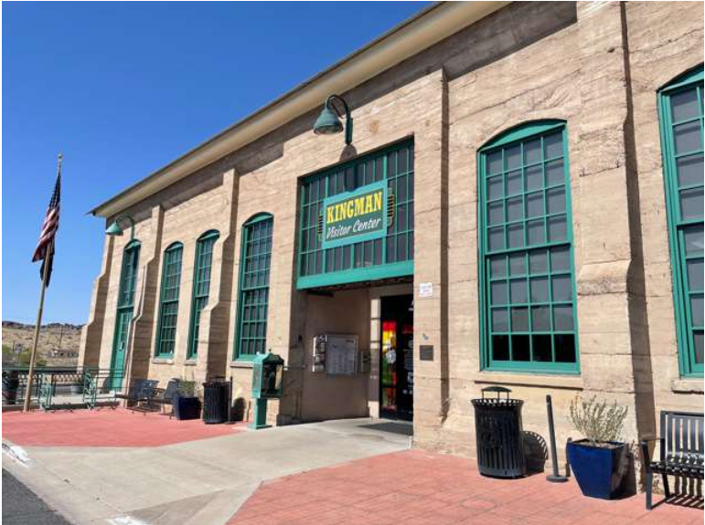
Title: Powerhouse Visitor Center
