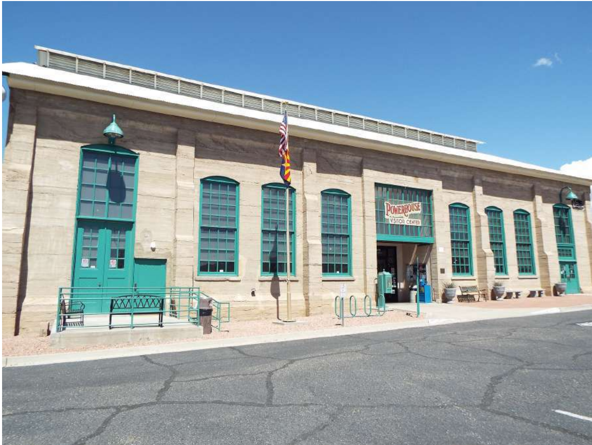
Image C-16: The Re-adapted Powerhouse, Kingman, Arizona
