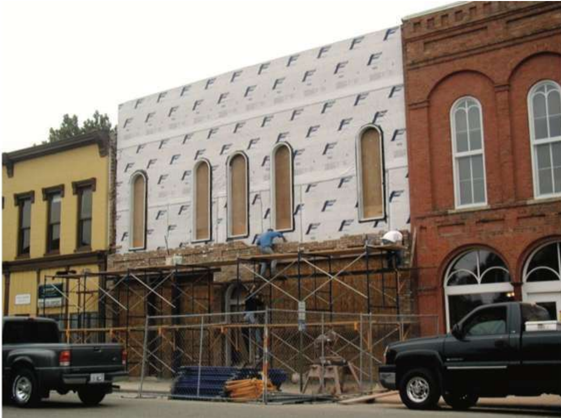
Image C-4: The Palms Grill Café during the restoration process
